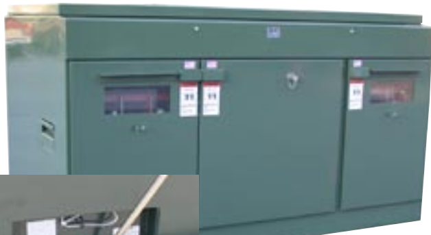
Figure 1b. Unit pictured with security window covers removed. Inset shows key interlock on switch handle that sequences access to key interlock on metering compartment door.
