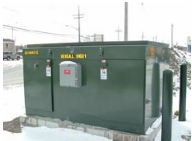
Installation views of primary metering unit shown with customer installed (on center compartment doors) kilowatt-hour meter (in green box) and key interlock transfer block (in gray box) for the connected distribution transformers.
