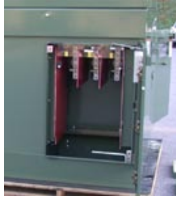
Figure 5. Open door view of incoming bus-termination compartment with bus connecting to top terminals of switch and allowing switchblades to be de-energized (if no backfeed from the load circuit) when the switch is open.
