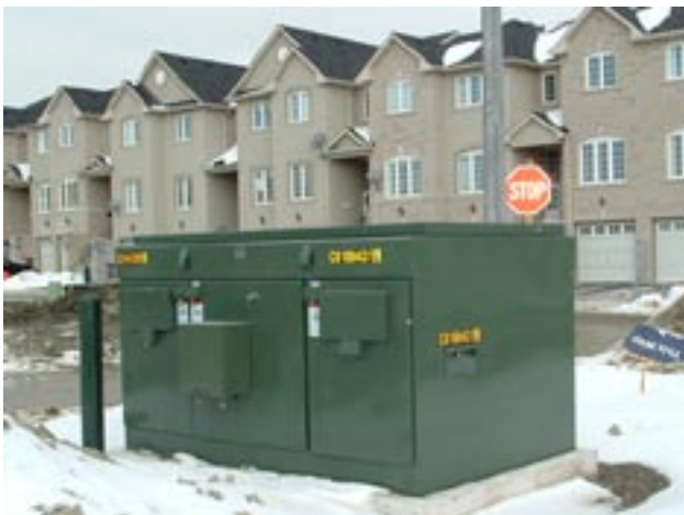
Installation views of primary metering unit shown with customer installed (on center compartment doors) kilowatt-hour meter (in green box) and key interlock transfer block (in gray box) for the connected distribution transformers.
